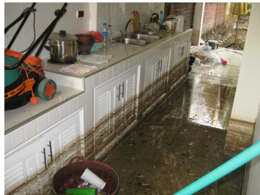
Fig. 4. Water level inside a house (Nov.26 th , 2011)
